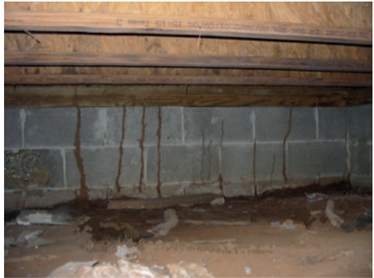
FIGURE 4. Inspection areas and evidence of subterranean termites (mud tubes)
