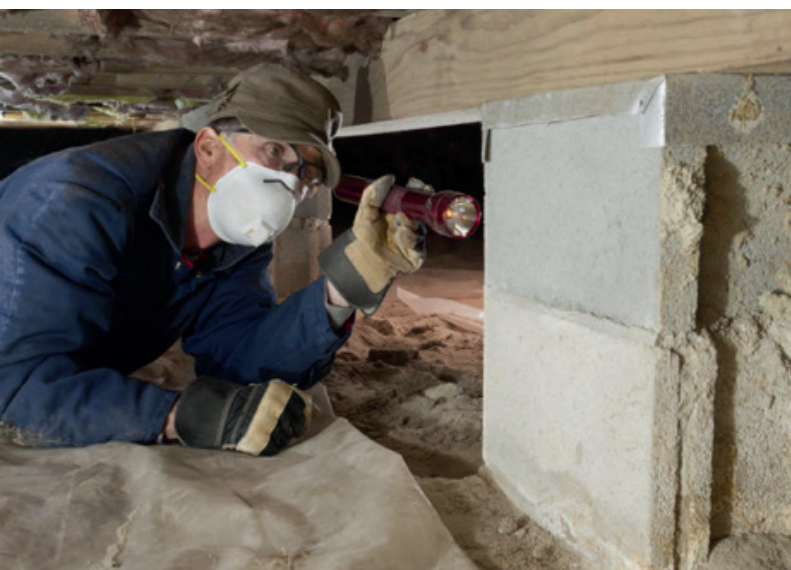
FIGURE 3. Visual termite inspection
