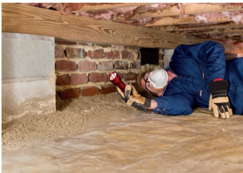
FIGURE 3. Visual termite inspection
